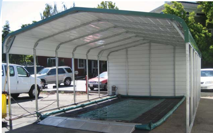
Porta-Pad installed with Canopy and Additional Ramping.
